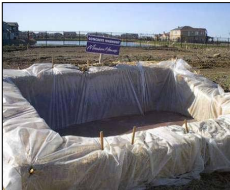
Plate 3-1 Typical concrete shoot wash out areas
